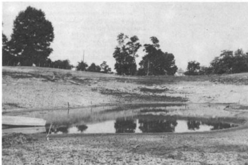
The Brumagen pond collapse (summer 1978), just after failure occurred. The pond has not been reestablished and today is filled with brush and small trees. Photo by Gary O'Dell.
