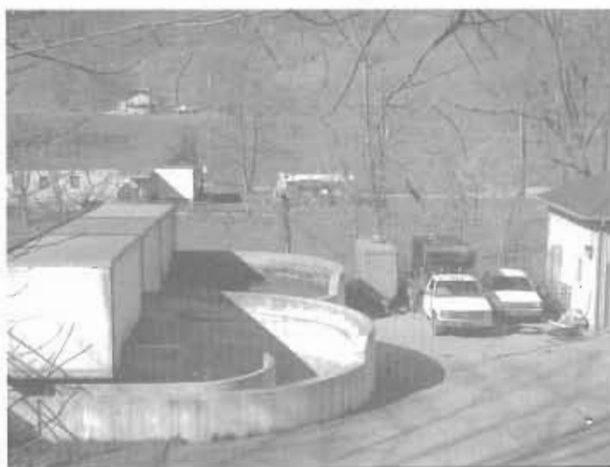
The ironies of uneven development: across the creek from the Fleming-Neon sewage treatment plant in Letcher County, mobile homes discharge raw sewage directly into Boone Fork Creek through straightpipes.
