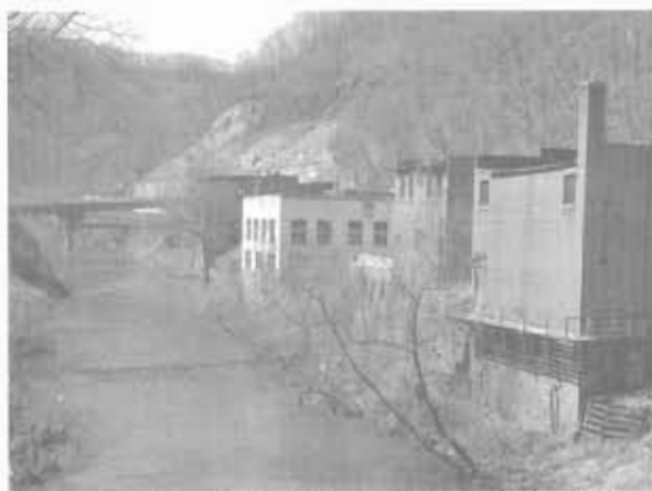
The "back side" of Iaeger, WV, viewed from the Tug Fork. Before the public system was acquired by the McDowell PSD in 1999, the water here was unsafe to drink. All photos by Gary O'Dell
