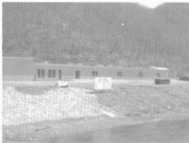
The only water supply for this new Sandy River Middle School in McDowell County was well water contaminated with salt brine.
