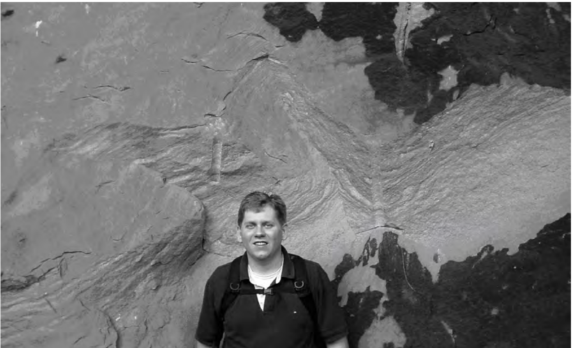
FIGURE 6. Drill holes and associated spalling along the rear wall of the JFB Niter Mine (15WO21) in Wolfe County. (Photo by Gary O'Dell, 2004.)
