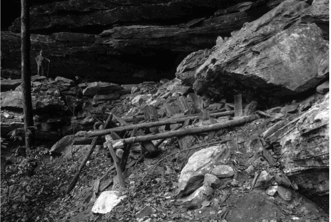
FIGURE 7. Two Type I leaching vats in the Trinity Niter Mine (15WO206) in Wolfe County contained within a pole framework 3 m deep and 3.7 m wide. (Photo by Fred E. Coy, ca. 1982.)
