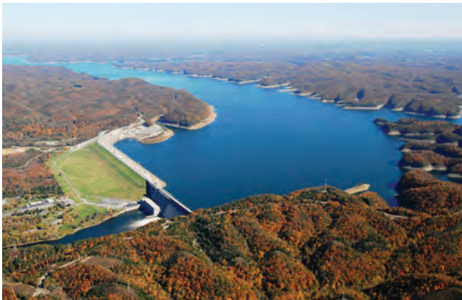
Wolf Creek Dam and Lake Cumberland. Photograph was taken in November 2009 when lake level had been reduced to investigate and remediate serious bypass leakage. Regional cavers took advantage of the reduced pool to explore Crystal Cave passages. Source: USACE.
