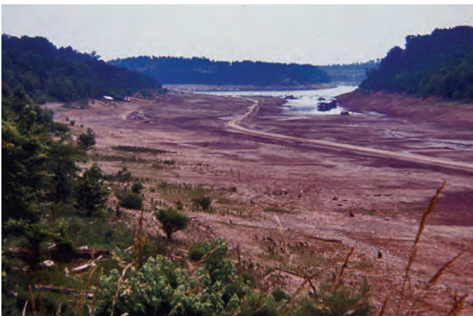
During the summer of 1968 the water level in Lake Cumberland was reduced by 40 feet to address bypass leakage around Wolf Creek Dam, exposing the valley bottom east of Burnside Island. The community of Burnside was formerly situated in this valley and was relocated to the north. Visible in the photograph is old Highway 27, also relocated, with stranded boat docks in the background and the channel of the Cumberland River in the distance. The temporarily reduced pool level allowed cavers to enter Rock Sink and explore part of Crystal Cave. Photo: Gary A. O'Dell, 1968.
